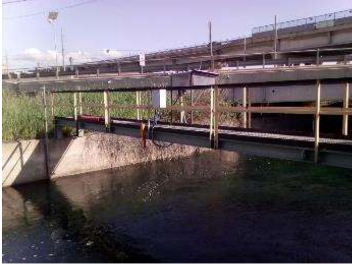
I/va, water discharge, Steel Factory
